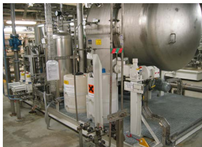
Figure 1.1: Potable water system with evaporator, scale inhibitor tank, chlorine tank, alkalising filter and UV units (Photo: Eyvind Andersen)
