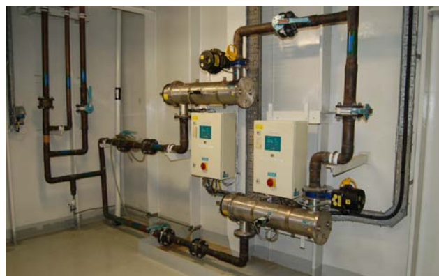
Figure 8.5: This UV unit has two radiation chambers, each with a control panel (white) and an UV sensor (on the front). The black valve closes if the radiation falls below the alarm level. (Photo: Eyvind Andersen)
