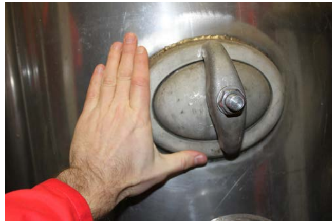
Figure 5.5: Alkalising filters, hydrophore tanks and calorifiers are often supplied with access openings of such a small size that the tanks are impossible to clean (Photo: Eyvind Andersen)
