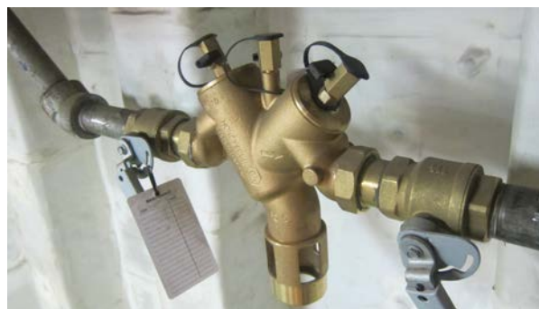
Figure 9.17: If other liquid carrying systems must be supplied with pressurised potable water, a BA type backflow prevention device gives the best level of protection. Note the 3 test points on top of valve. This valve needs to be fitted with a strainer and stop valves before and after for testing, and location over a drain is recommended, as it may open automatically (Photo: Eyvind Andersen)
