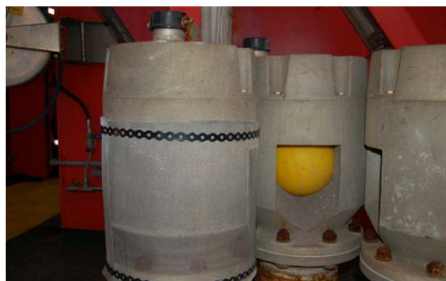
Figure 9.3: Protect air vents for potable water tanks. The picture shows vents safeguarded with floating ball and fine mesh corrosion material. The picture is taken on a newbuild prior to marking (Photo: Eyvind Andersen)
