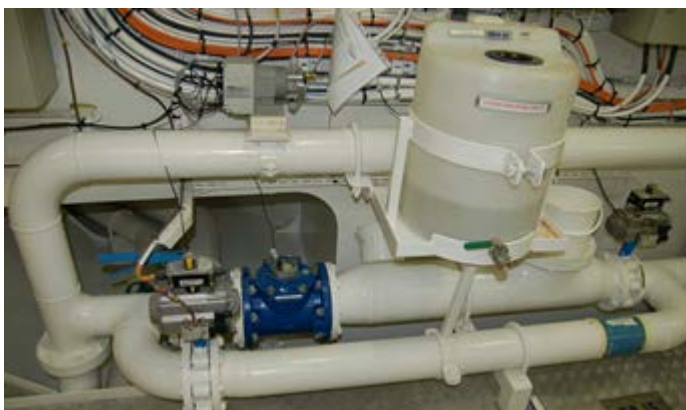
Figure 8.3: Flow meter-controlled chlorination unit (Photo: Eyvind Andersen)
