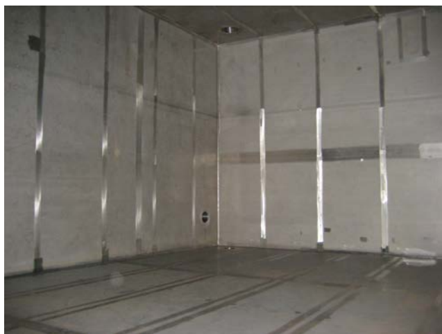
Figure 9.1: Approximately 4 metres high potable water tank in stainless steel with no obstructing internal structures. Such tanks are easy to clean, with no problems with applying and maintenance of coating (Photo: Bjørn Løfsgaard)
