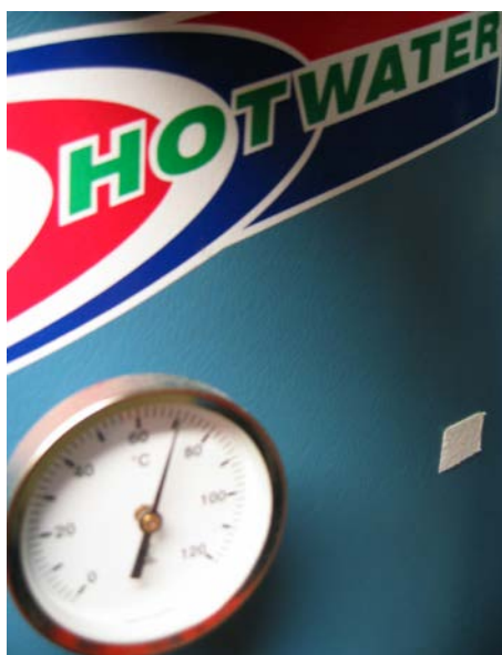
Figure 9.21: Legionella can be prevented by keeping the cold water cold and the hot water hot (Photo: Eyvind Andersen)
