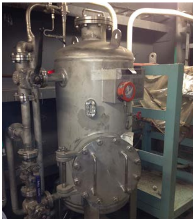
Figure 9.6: Also smaller tanks in the potable water system, like hydrophore tanks, calorifiers and alkalisng filters must have sufficient access for inside maintenance. The pictured tank is made of stainless steel and has sufficient manholes (Photo: Eyvind Andersen)
