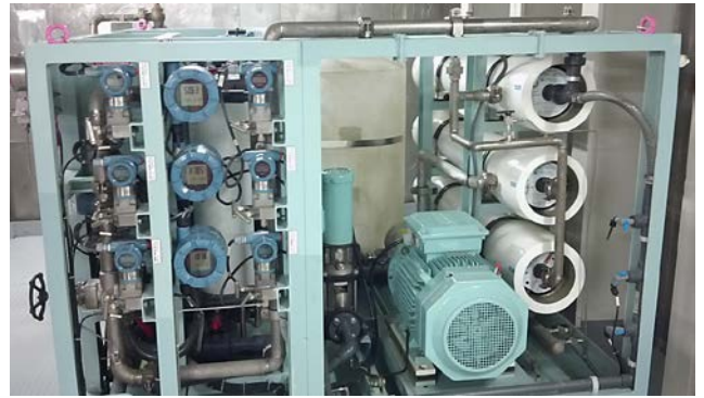
Figure 6.7: Reverse osmosis unit. The membranes lay coiled within the white tubes on the right (Photo: Eyvind Andersen)
