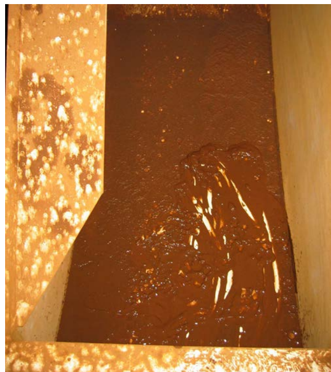
Figure 3.1: The requirement to clean tanks at least once a year is intended to avoid the situation shown above, where there is a layer of mud at the bottom of the tank. This must be handled as a non-conformity case. (Photo: Bjørn Løfsgaard)
