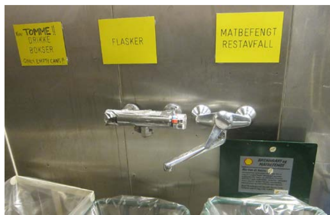
Figure 9.22: A sink has been removed whilst pipes and fittings remain, leaving dead ends where Legionella may have good growing conditions and later infect the rest of the potable water system (Photo: Eyvind Andersen)
