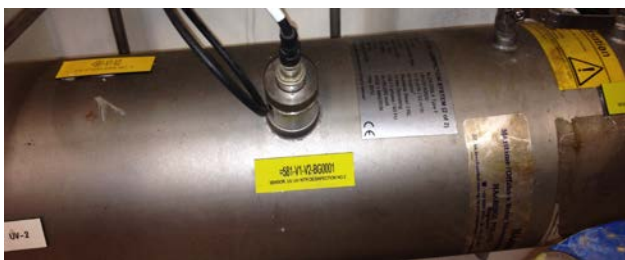
Figure 8.8: Here, the UV sensor is placed on top of the UV chamber (Photo: Eyvind Andersen)
