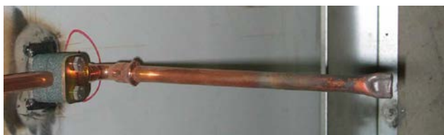
Figure 5.2: During the construction process it is important that pipe systems are not contaminated. The picture shows how pipe ends are secured by compression (Photo: Bjørn Løfsgaard)
