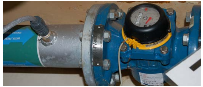
Figure 7.7: The flow meter display is visible to the right, and the chlorine hose and dosing point to the left (Photo: Eyvind Andersen)
