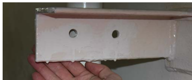
Figure 9.11: Picture from a tank where incorrect coating has resulted in corrosion and need for touch ups. Coating applied wrongly and too thick on cold steel increases the risk for microbial growth, and may cause unpleasant odour and taste from tank coating (Photo: Eyvind Andersen)
