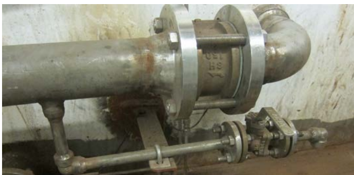
Figure 9.14: This test tap is not designed correctly, as it is too long and too big. In addition the outtake below the main pipe will increase the risk of biofilm formation, as dirt and particles will settle in the test pipe, and the water tests may not be representative (Photo: Eyvind Andersen)
