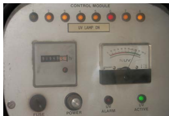
Figure 8.9: Control panel for UV unit with eight UV lamps. As both tube 6 and the signal lamp for tube 1 is defect, the UV unit is unsafe. The UV intensity is still quite high. This may be due to clear water or long distance between UV sensor and the defect UV lamp (Photo: Eyvind Andersen)
