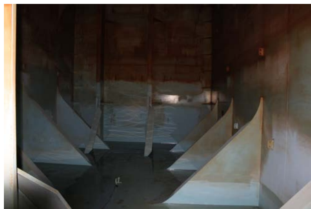
Figure 5.3: This potable water tank is high and lacks internal platforms for easy cleaning. This has resulted in insufficient cleaning. The walls are clean up to 2 metres and very dirty above 4 metres (Photo: Eyvind Andersen)
