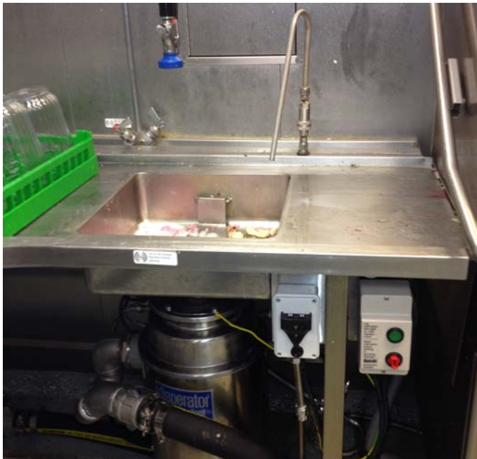
Figure 9.16: Full air gap of type «AA» is the best way of eliminating contamination from other systems supplied with potable water. Here water is supplied to a food grinder via pipe above the sink to the right (Photo: Eyvind Andersen)
