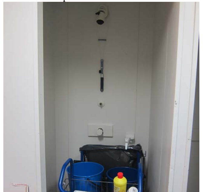
Figure 9.13: This shower is not in use, and is used for storage. Water in such pipes will be at room temperature, and there is a growth potential for Legionella and other microbes. This water may then contaminate the rest of the piping. Piping that is not in use should be eliminated, alternatively flushed weekly (Photo: Eyvind Andersen)
