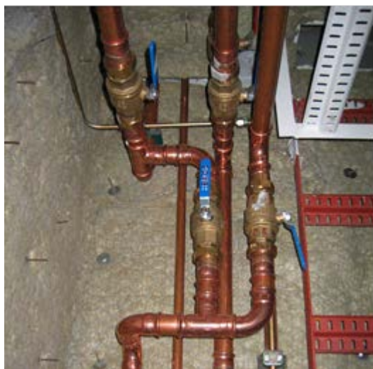
Figure 4.7: Corrosive water in copper pipes can result in excessive copper content in the potable water (Photo: Bjørn Løfsgaard)
