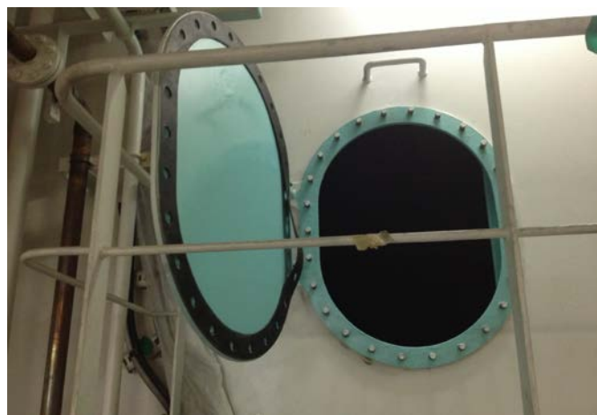
Figure 9.5: The picture shows a storage tank with an accessible manhole (Photo: Eyvind Andersen)
