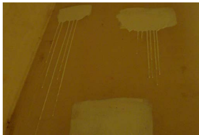
Figure 9.10: Incorrect coating. A roller has been used instead of a round brush, and the coating has been used on too large areas and in a far too thick layer (Photo: Bjørn Løfsgaard)
