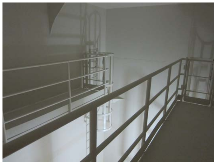
Figure 9.2: Access platforms aid maintenance in tanks over 4 metres high. Internal structures in tanks should be minimised to enhance circulation and minimise maintenance. Circulation is achieved by placing the inlet in one upper corner of the tank, whilst the outlet is placed in the opposite lower corner (Photo: Eyvind Andersen).
