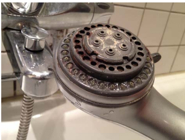
Figure 9.24: Such biofilm is a consequence of insufficient cleaning. Microbes have ample possibility for growth (Photo: Eyvind Andersen)
