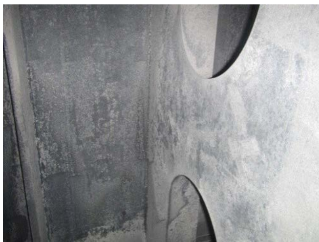
Figure 9.7: «White rust» in a potable water tank, is deposits of zinc carbonate. The tank is coated with a product that contains zinc, and that can be used in the pH interval 5.5 to 10. At higher pH, problems with deposits and high zinc levels in the water can occur. In this case poor pH management is the source of the problems, as the measured pH around 11 was far beyond the max limit of 9.5 in the potable water regulations. (Photo: Tjarda den Dunnen)
