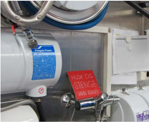
Figure 9.19: A hose station where water is leaking between the hot and the cold water when the mixer is left in open position and the hose is not in use. A sign to close the mixer is not a barrier against such leaks (Photo: Eyvind Andersen)
