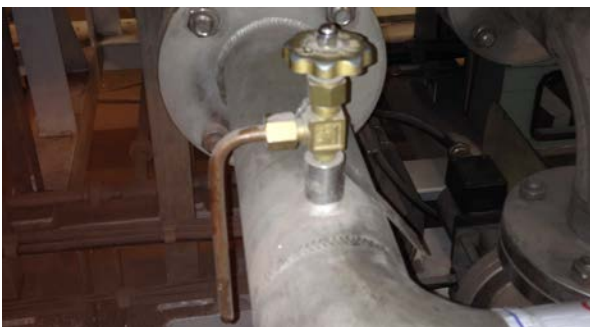
Figure 5.8: Short and self-draining test tap with sufficiently small pipe diameter. The short distance from main pipe to valve eliminates stagnant water. By placing the outtake on the upper half of the pipe, trapping of particles is avoided. A shorter sample point end would have eased sample point disinfection (Photo: Eyvind Andersen)
