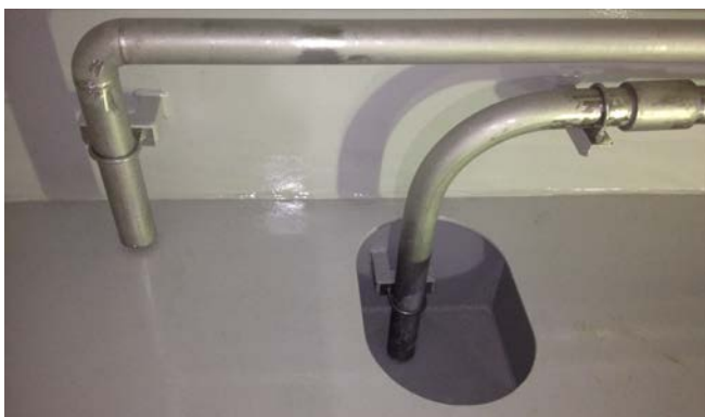
Figure 9.4: Tank suction (left) is elevated a few centimetres from the tank floor, whilst a drain suction pipe in the pump well in the middle makes it easy to empty the tank (Photo: Eyvind Andersen)
